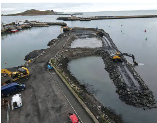
Construction of bunded area for dredge spoil
