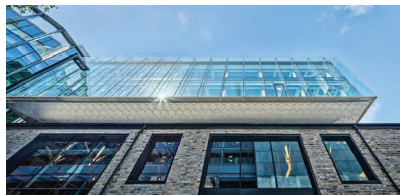
View of completed Block 2, 'floating' over the warehouse. Photograph taken from internal landscape courtyard
