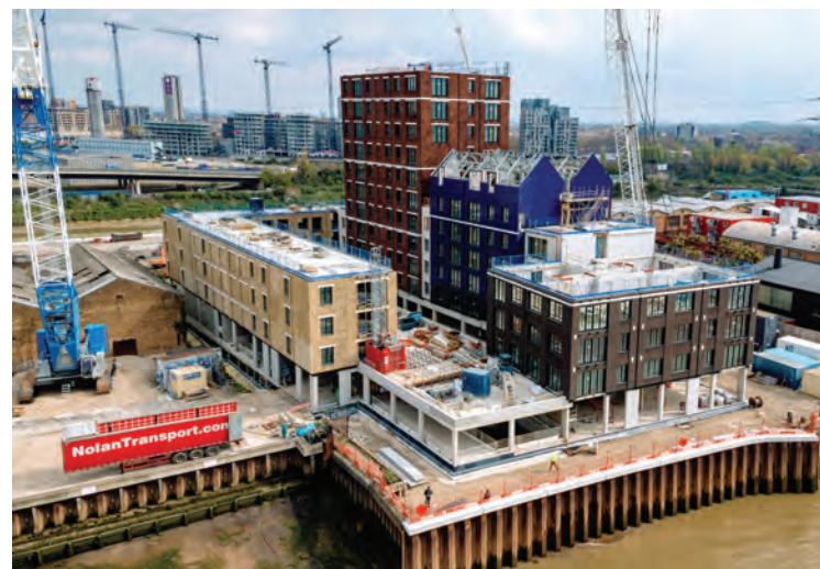
Block JKL under construction
