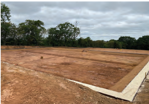
Earthworks and construction of the ponds
