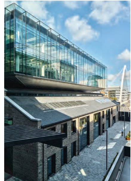
View of completed Block 2, 'floating' over the warehouse. Photograph taken from Block 1
