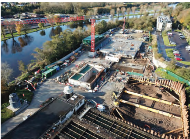
Lee Road Water Treatment Plant under construction
