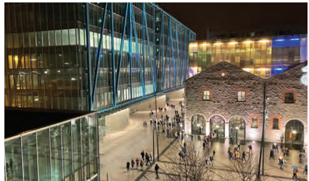
The external lighting design for both the EXO and the Point Square was carried out by OCSC. The lighting design included the upgrade of the CCTV and security systems
