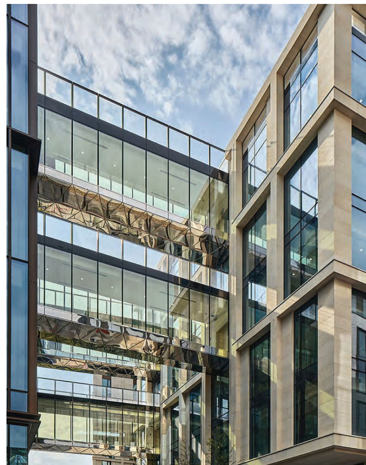
Link bridge between buildings
