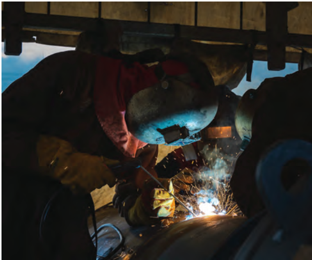
Welders working on a 900mm pipe
