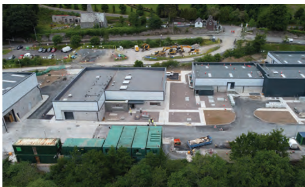
Lee Road Water Treatment Plant exterior view
