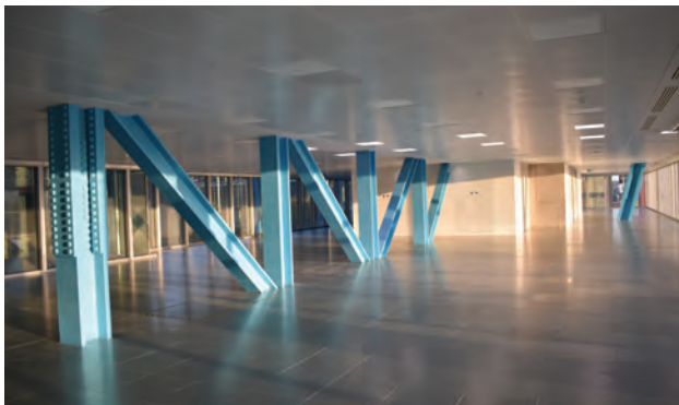
1st floor transfer truss and diagonal megacolumn
