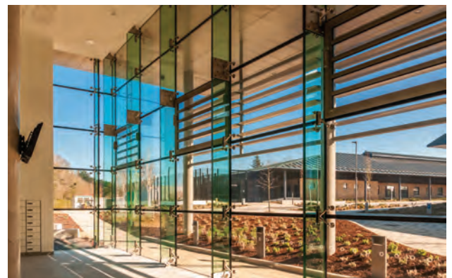
View from Reception Building towards ICRU Building
