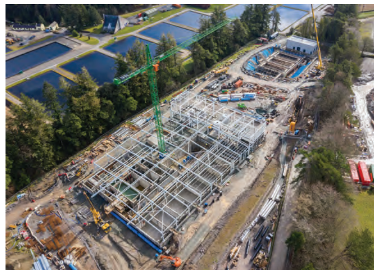
Vartry Water Treatment Plant under construction alongside existing slow sand filters
