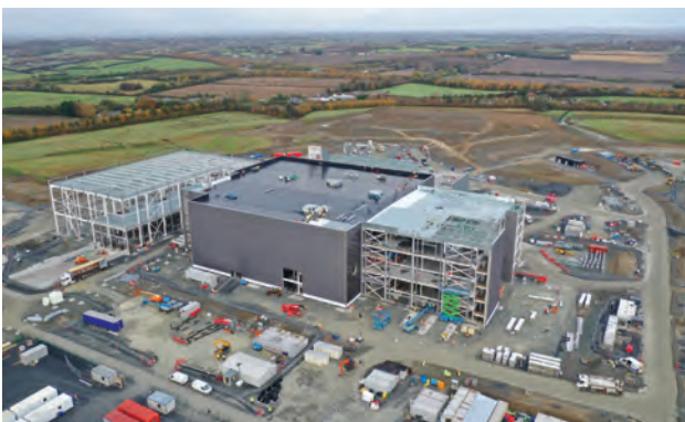
Aerial View – WuXi Biologics under construction
