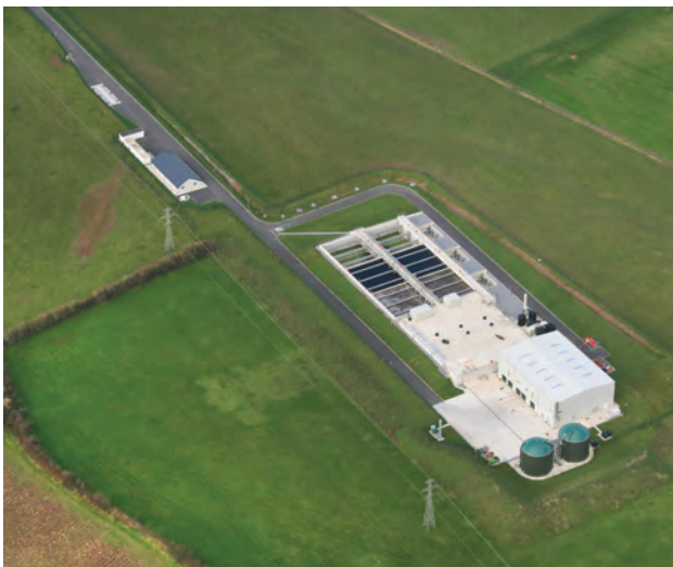
2022 – Project of the Year: Nicholas O'Dwyer Limited, Cork Lower Harbour Main Drainage Scheme
