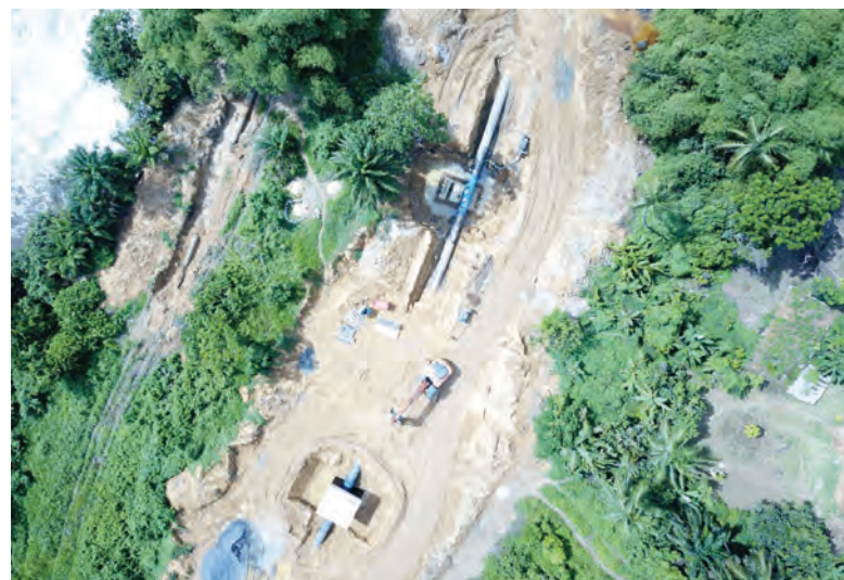
Drone photography was used on a regular basis to monitor progress
