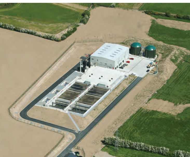
Overview of the WWTP – the use of Nereda® technology resulted in the footprint of the 65,000PE WWTP being relatively small
