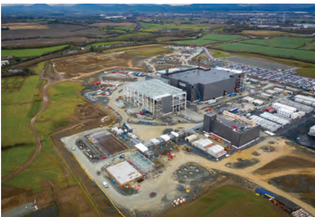
Aerial View – WuXi Biologics under construction
